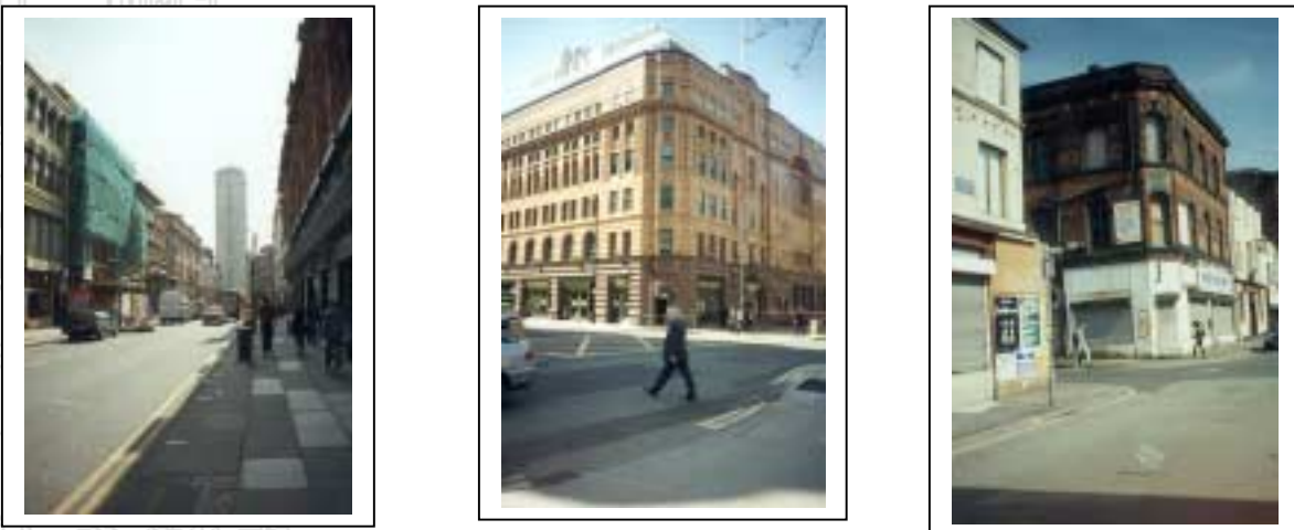
Figure 4.13 The Rebuilding Continues: Source: G.W. Dickson
