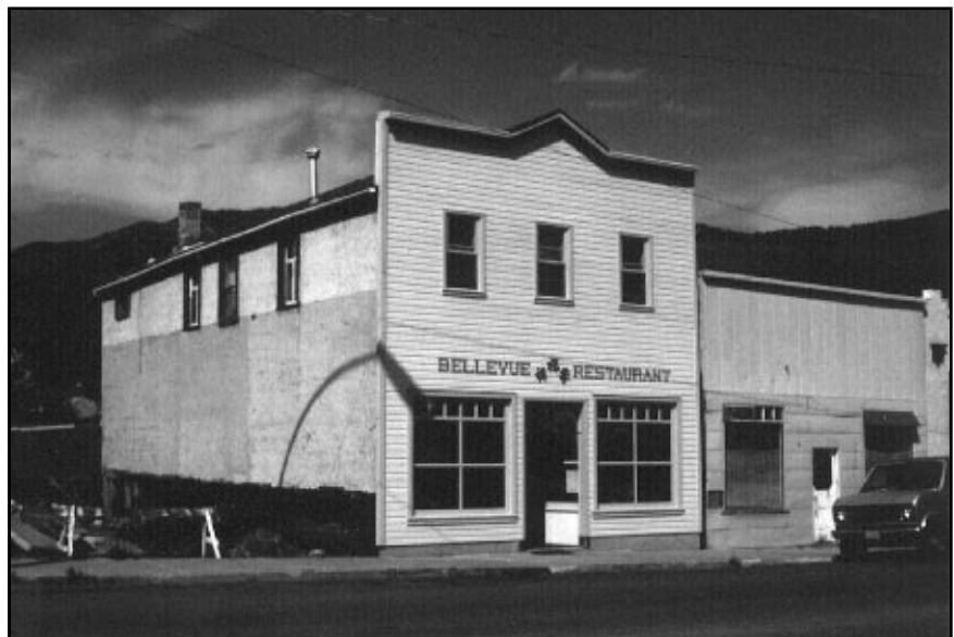
Rehabilitated Main Street building in Bellevue
