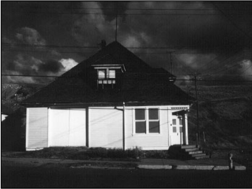
Rehabilitated building in Coleman
