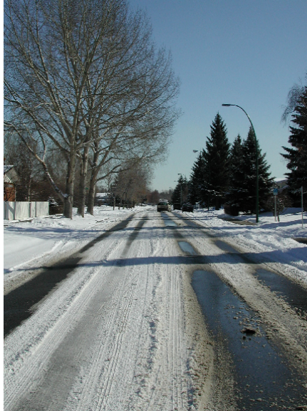
Figure E.8: Capri Avenue Looking Southwest
