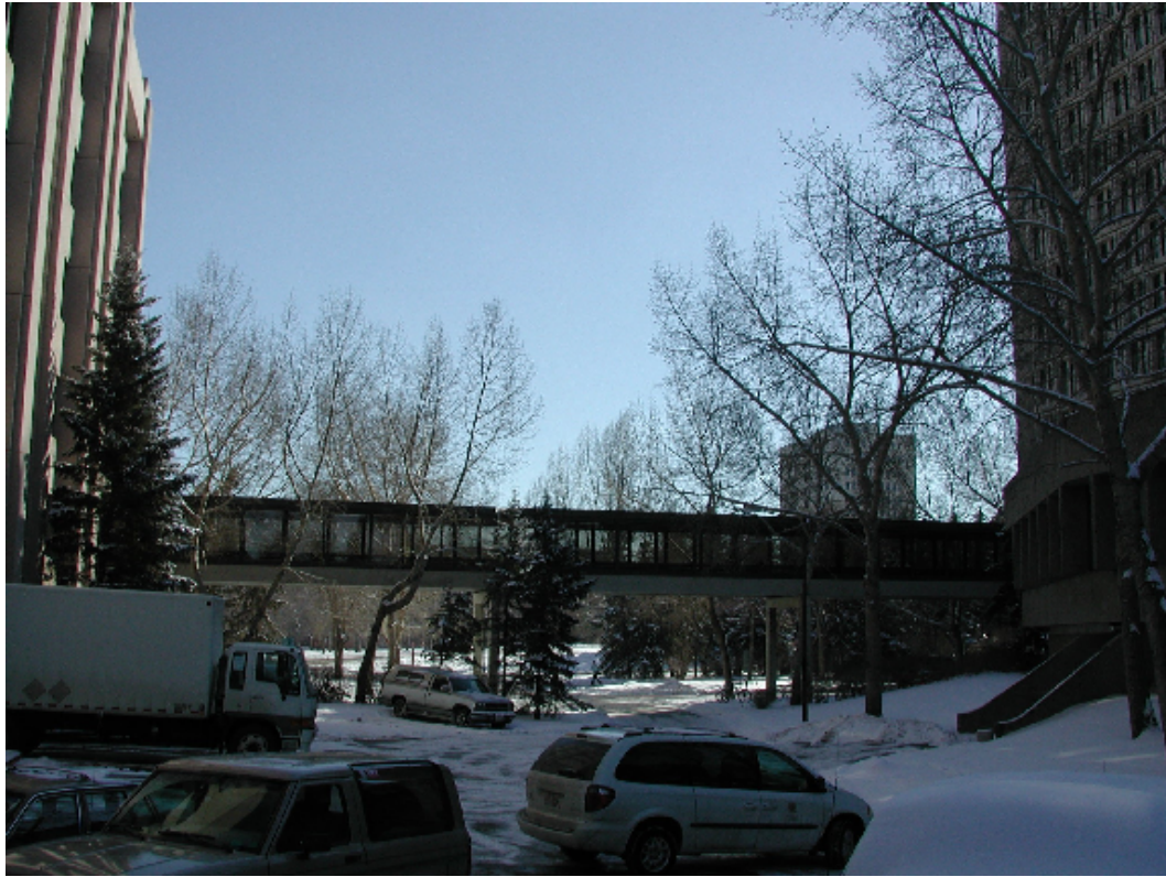
Figure 8.9: Point “B” Looking South
