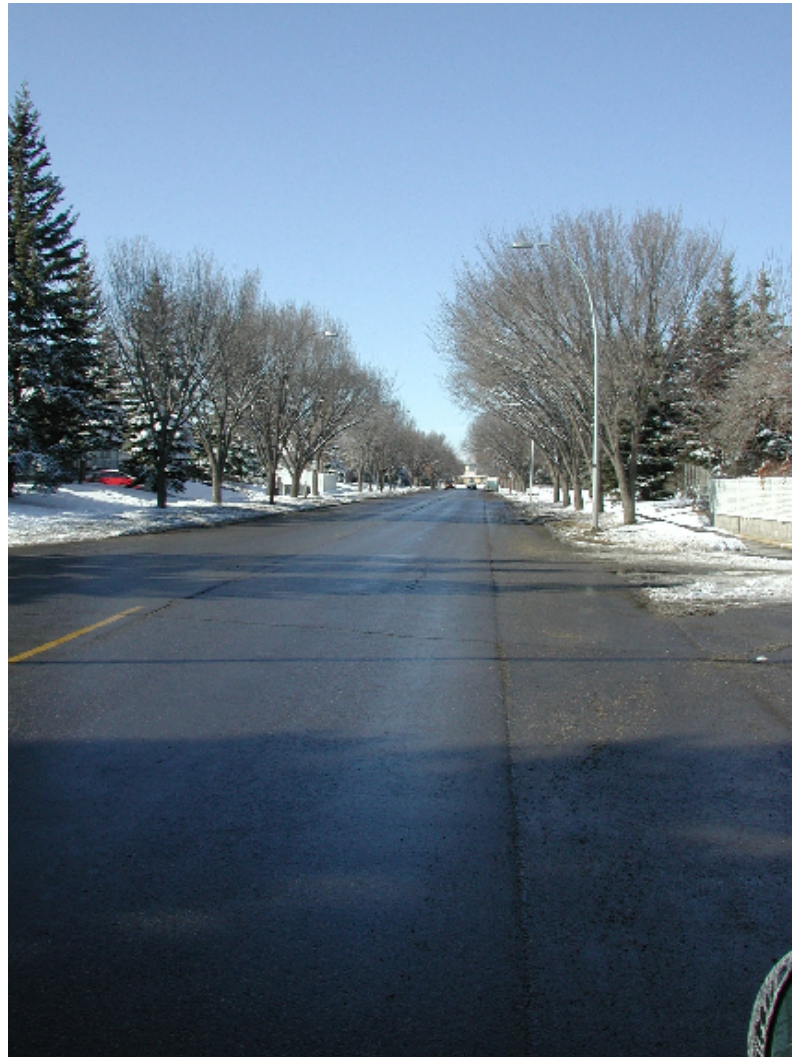
Figure 8.2: Northland Drive Looking Northwest
