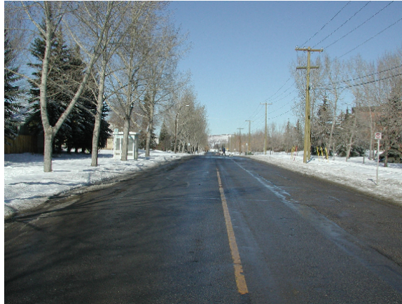
Figure F.2: 37 Street Looking North
