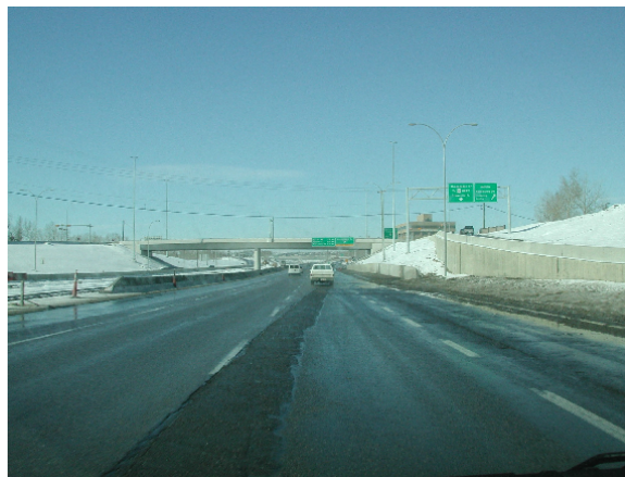
Figure E.11: Crowchild Trail Looking Northwest at Northland Drive Overpass
