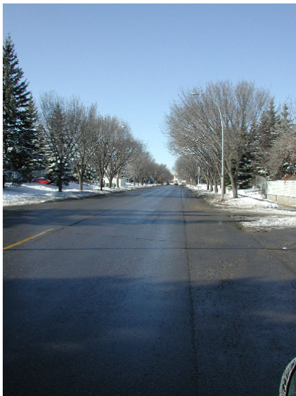
Figure E.6: Northmount Drive Looking Northwest
