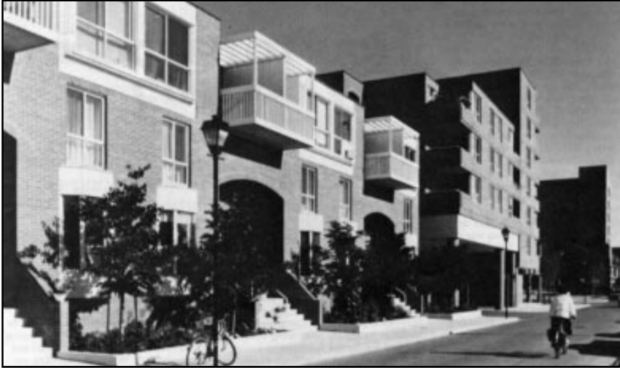
Figure 4: Toronto's traditional street system as seen by this street in St. Lawrence.
