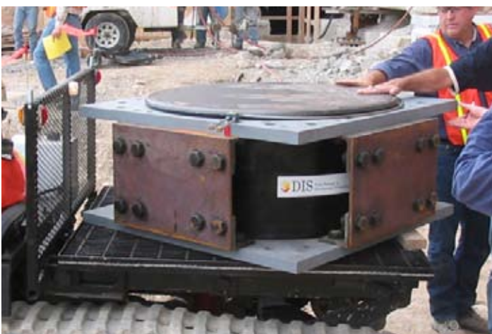
One of the 265 seismic base isolators.
