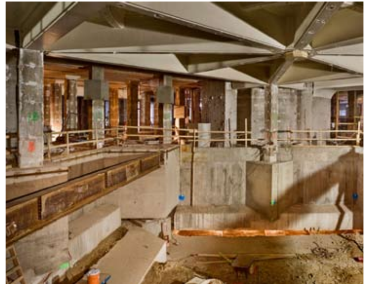
Rotunda load transfer during construction.
