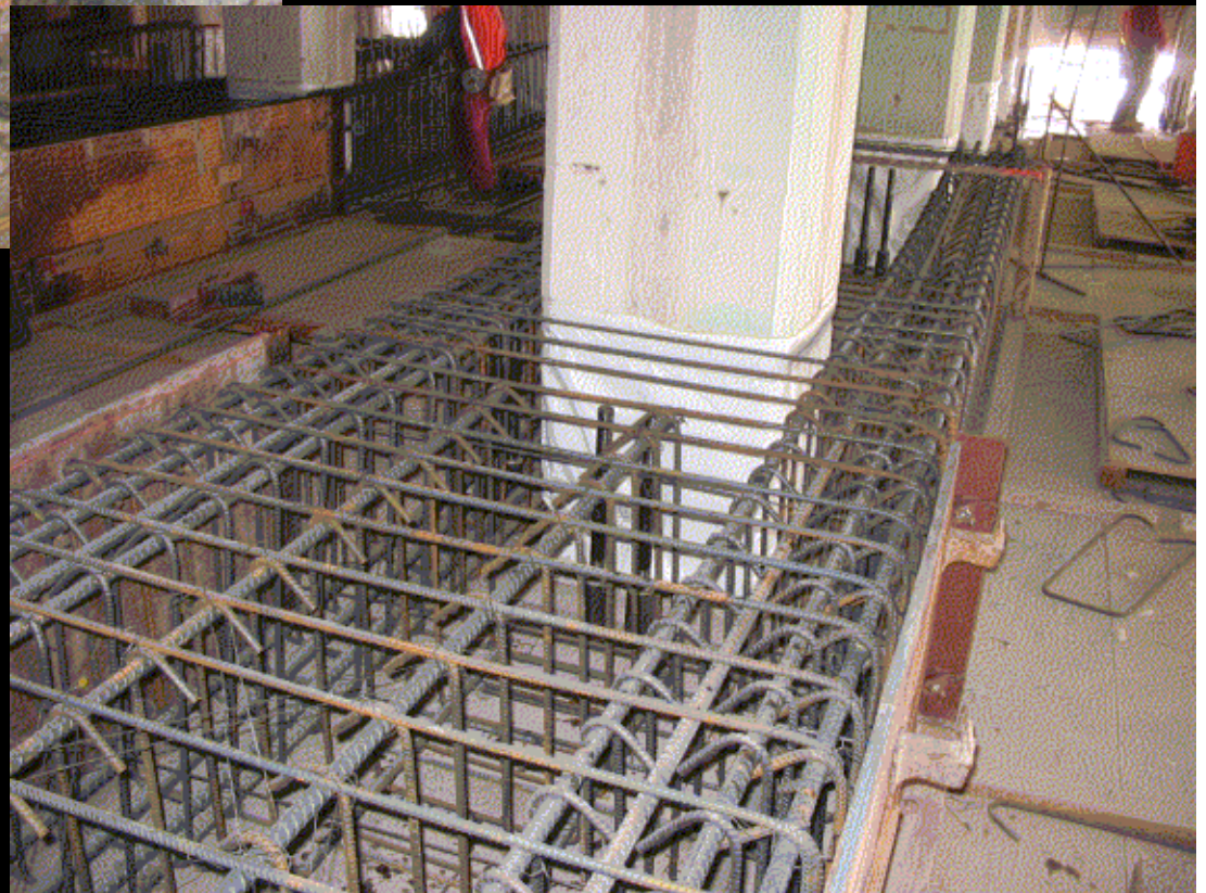
Assembly of Reinforcement
