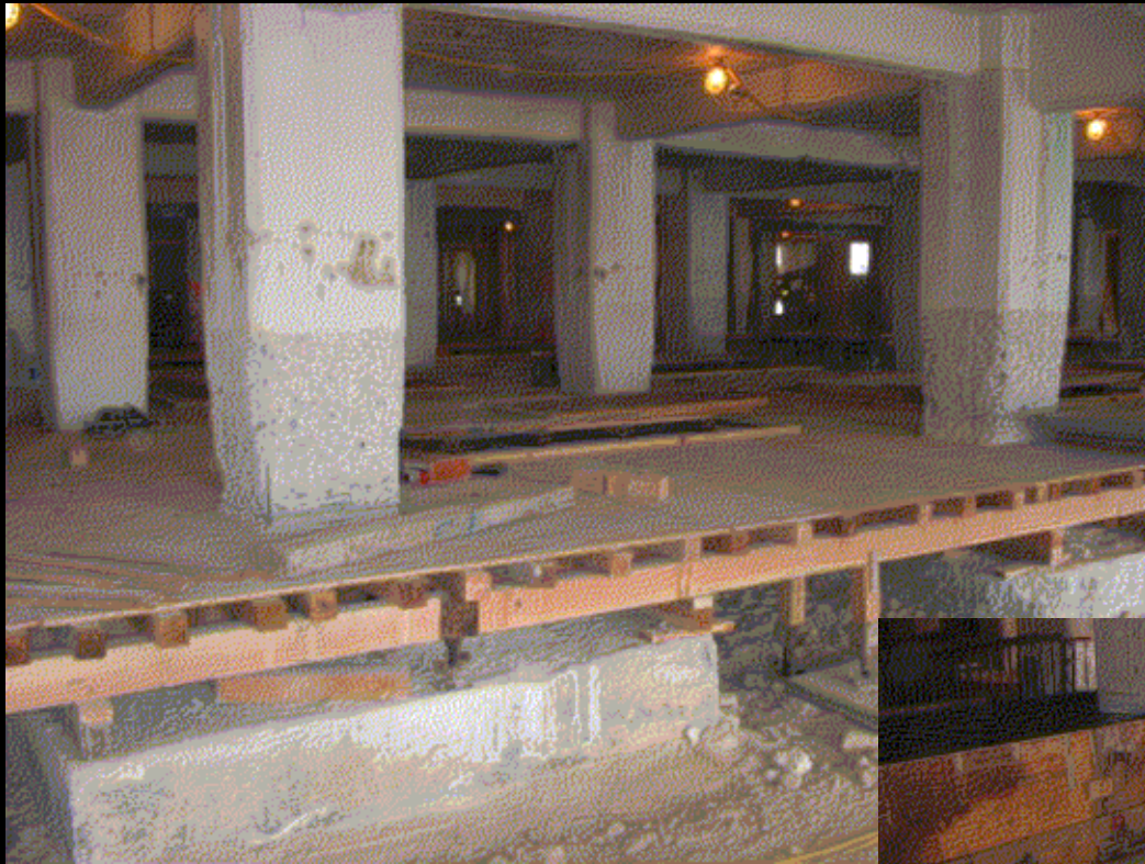
Assembly of Casting Deck
