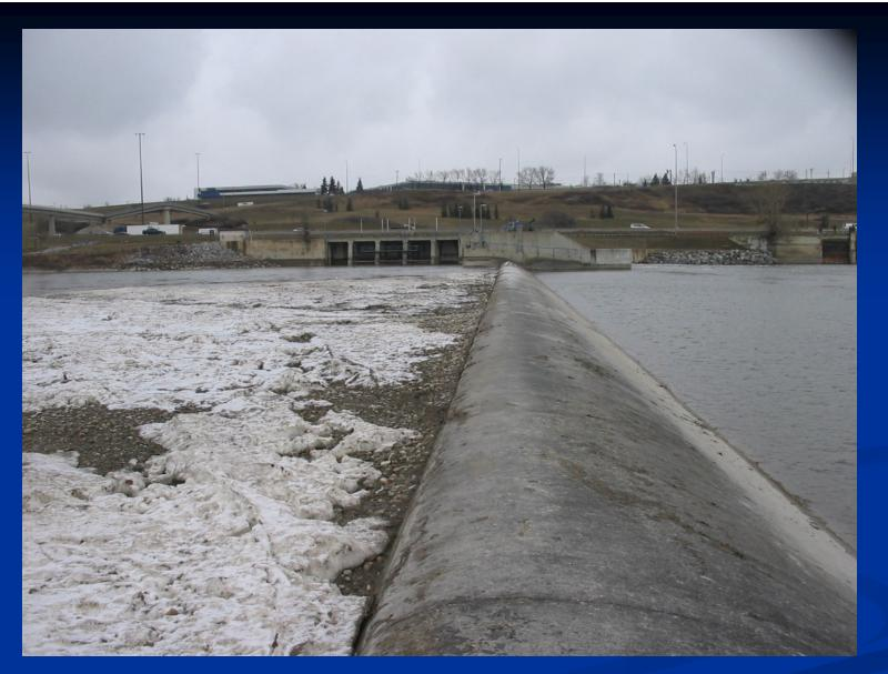
Existing Weir Looking Northeast (April 10, 2007) Note: Water Diverted Through Sluiceway
