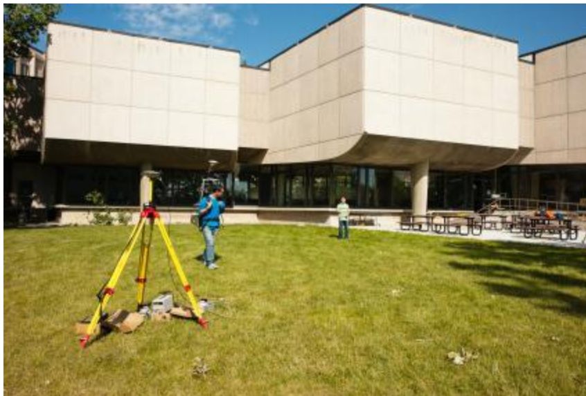
Figure 4.5: East Facing View of Engineering Lounge
