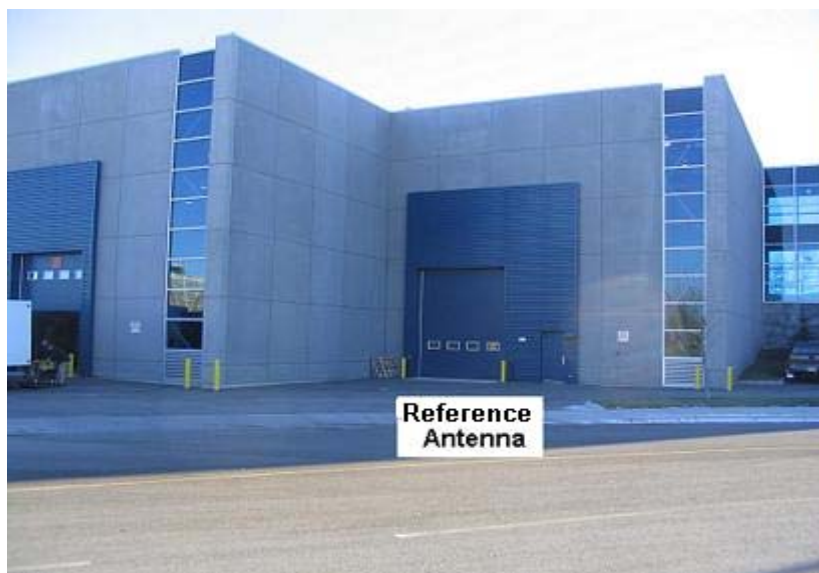
Figure 4.11: Surrounding Area for the Concrete Basement Test
