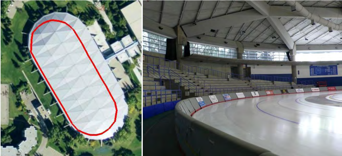
Figure 30 – Olympic Oval (Left: roof top with trajectory in red, Right: inside showing track and ice level)
